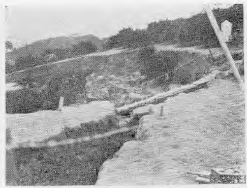
Fig. 1. Fissures on the south of Fūfuzuka.
