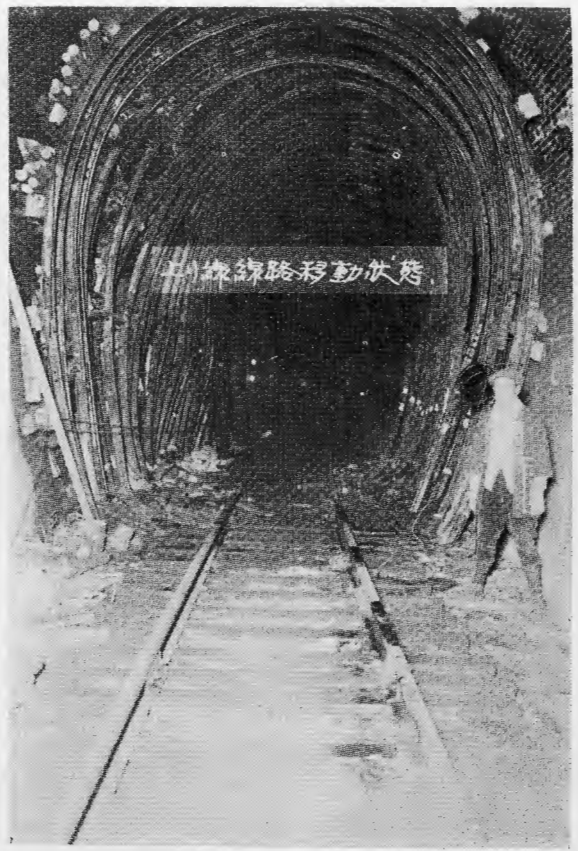
Fig. 1. Sifting and curving of the rail-center, up-track.
