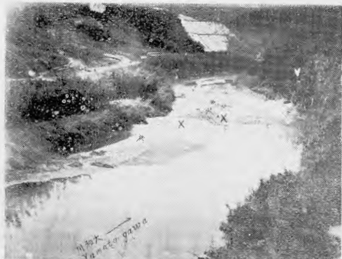
Fig. 3. Lifted river bed seen from a spot upstream. (Early in Feb.)
