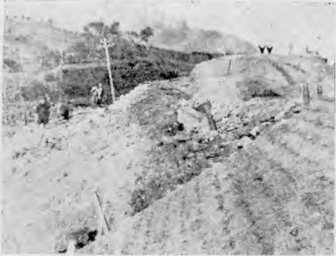
Fig. 4. Nearer view of the lifted part.
