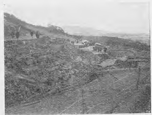
Fig. 2. Fissures on the south of seen from the west.
