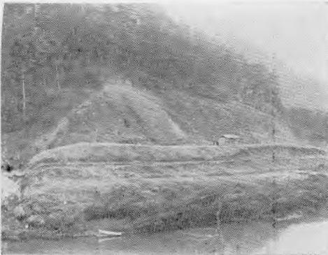
Fig. 3. Nearer view of the lifted part.
