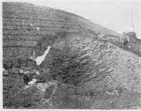
Fig. 4. Depression hole made on the south of Tōge village, just above the tunnel. The Tōge younger lava rich in platy joints.
