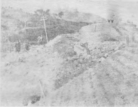
Fig. 4. Nearer view of the lifted part.
