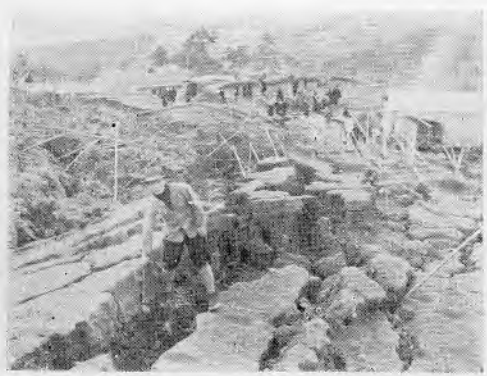
Fig. 3. The same as fig. 2. Internal view of the fissure.
