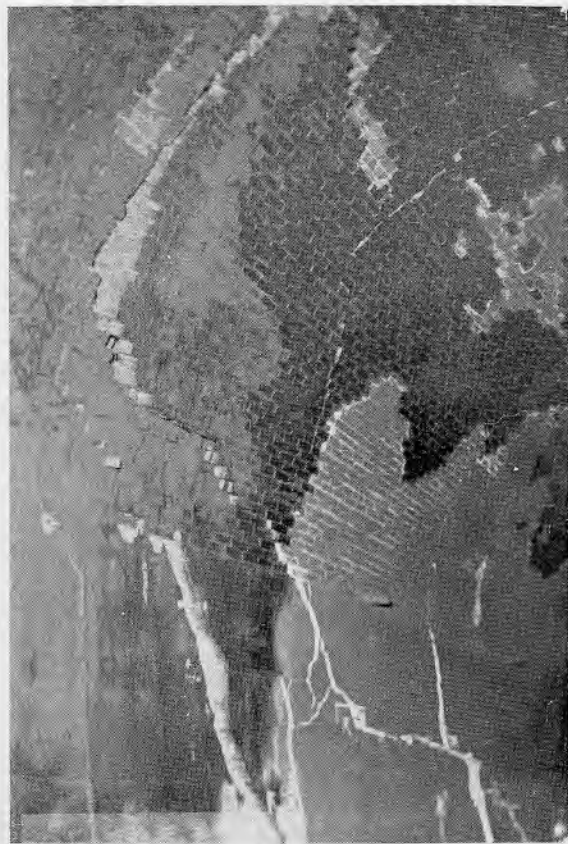
Pl. IX. Cracks appeared in the lining wall of the Kamenose tunnel, up-track. (Late in Jan.)
