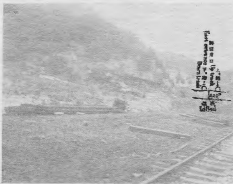
Fig. 3. Upheaval of the land to the west of the fissure shown in fig. 2, pl. IV. (Feb. 27)
