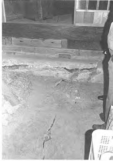
2. 民家の土台の右横ずれ変位 (Loc. 13) Right-lateral offset of the foundation of the house at Loc. 13.
