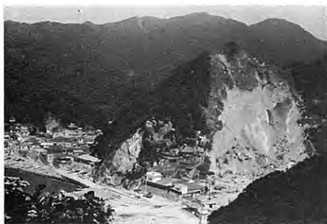
1. Landslide at Nakagi (loc. 68).
