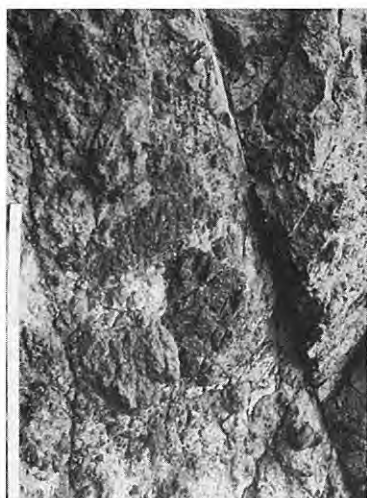
2. Exposed fault plane showing right-lateral slip at loc. I-1, east coast of Irozaki.
