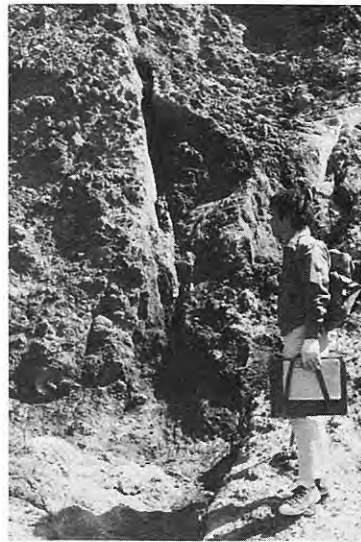
2. Faults at loc. 55.
