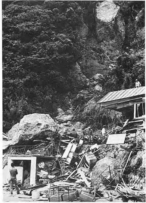
4. Complete collapse of a house caused by rock fall at Iruma.
