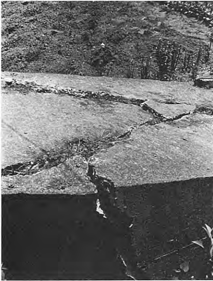
3. Damaged concrete road just on the fault line at loc. 6.
