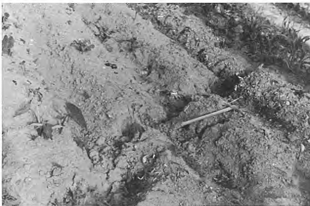
3. Damaged concrete road just on the fault line at loc. 6.
