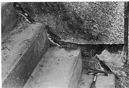
2. Right lateral displacement between steps and wall at the entrance of Isuzu Shrine (near loc. 47).
