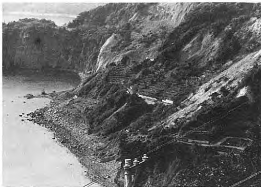
4. Debris and rock slides at 69 (this side), 79 and 80 (opposite).
