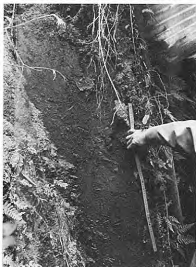
4. Exposed fault plane coated with thin fault gouge. Looking north at loc. I-3.
