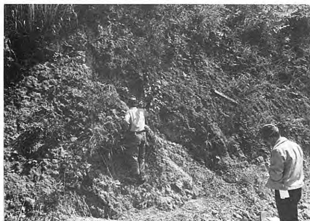
5. Slightly parted crack on bed rock at loc. 25.
