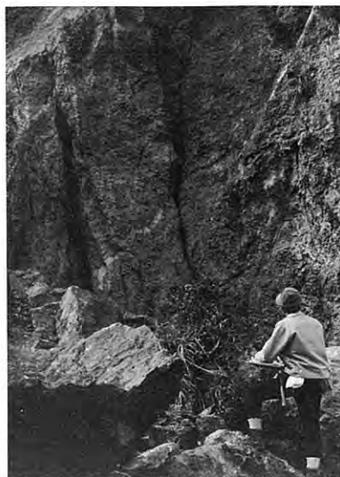
4. Open cracks at loc. 52.
