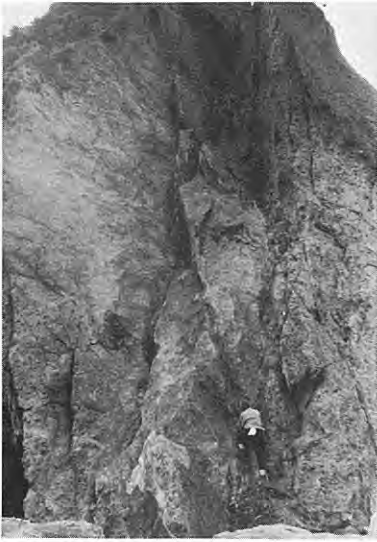
1. Faults and cracks at loc. 53. New exposure of slickensided fault plane (upper left part) was revealed due to collapse of the hanging wall.
