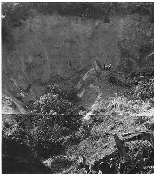
2. Landslide at loc. 68 (upper part).
