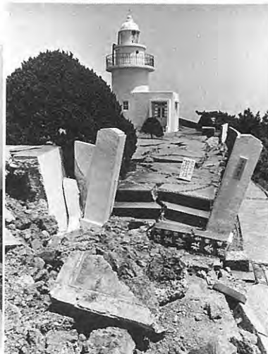
6. Damage to concrete road of Irozaki Lighthouse.
