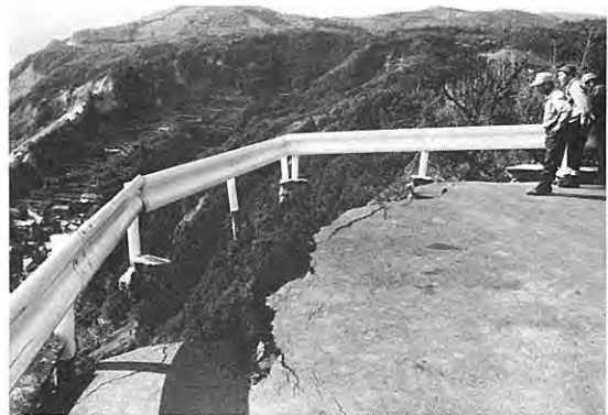
7. Lost foundation of a guard rail at loc. 77 and landslide topography at the upper part of Ochii Village.
