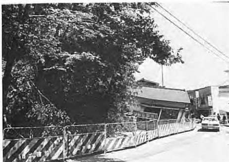
6. Destruction of a house caused by rock slide near loc. 72, Shimogamo.
