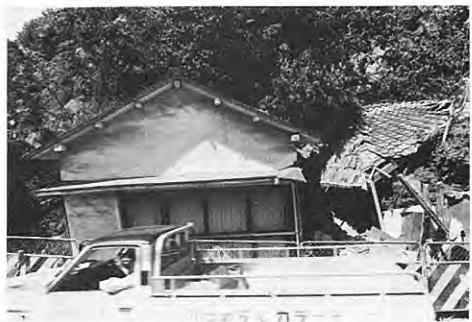
7. Damage to houses by rock slid at Shimogamo.
