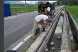
drilling in the firm concrete
