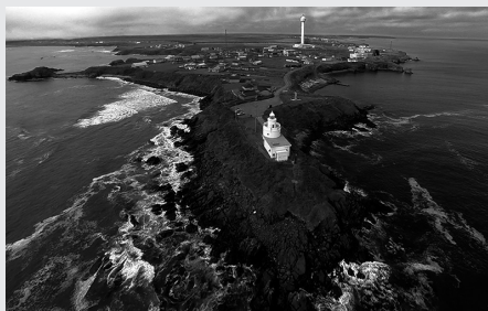
Aerial view of Cape Nosappu at the point of Nemuro Peninsular, eastern Hokkaido using an UAV.
