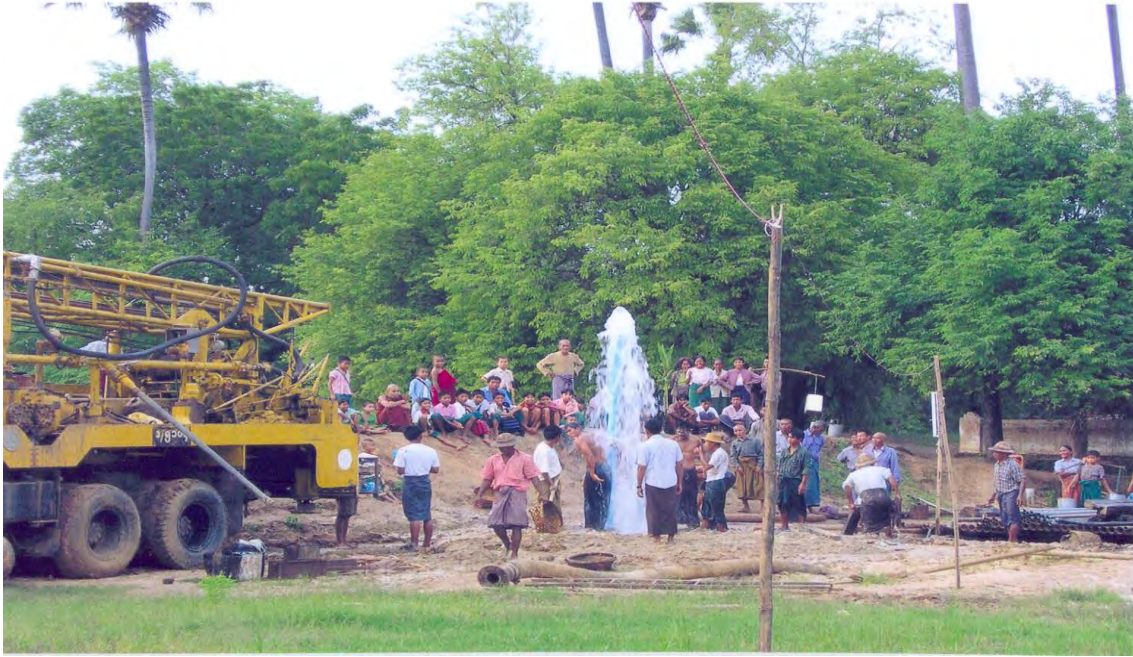
Fig. 8. Water Well Drilling Site (flowing tubewell at Sagaing Region)
