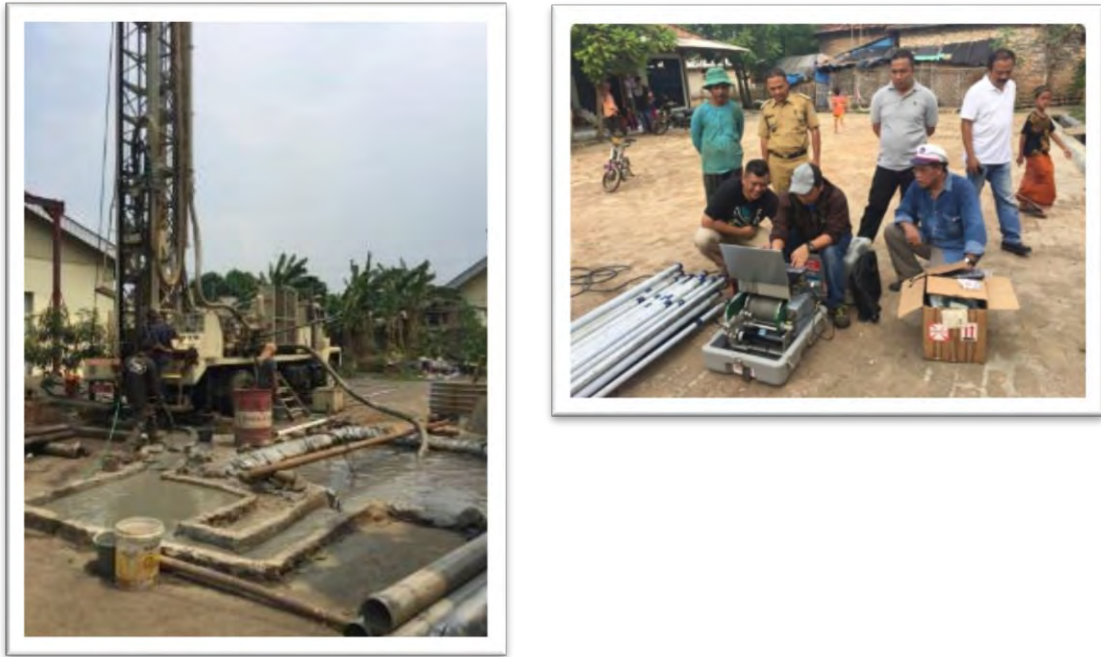
Fig. 6. Exploration drilling and well logging activities.
