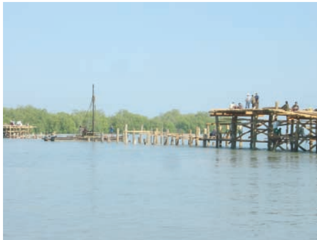
Photo 9. Destruction of wooden bridge to Plautonton by the tsunami.
