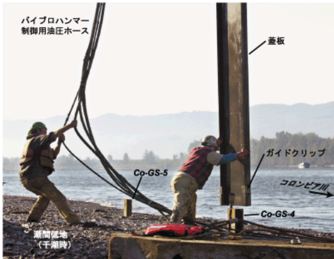
写真2. ジオスライサーふた板打込み作業 (Co-GS-4) . Photo 2. Driving the shutter plate along the sheet pile Photo by Bill Waguer, Longview Daily News.
